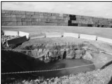
Boxes containing low-level radioactive waste lie in a shallow land burial trench. Alternative methods for the disposal of low-level waste are being developed.
